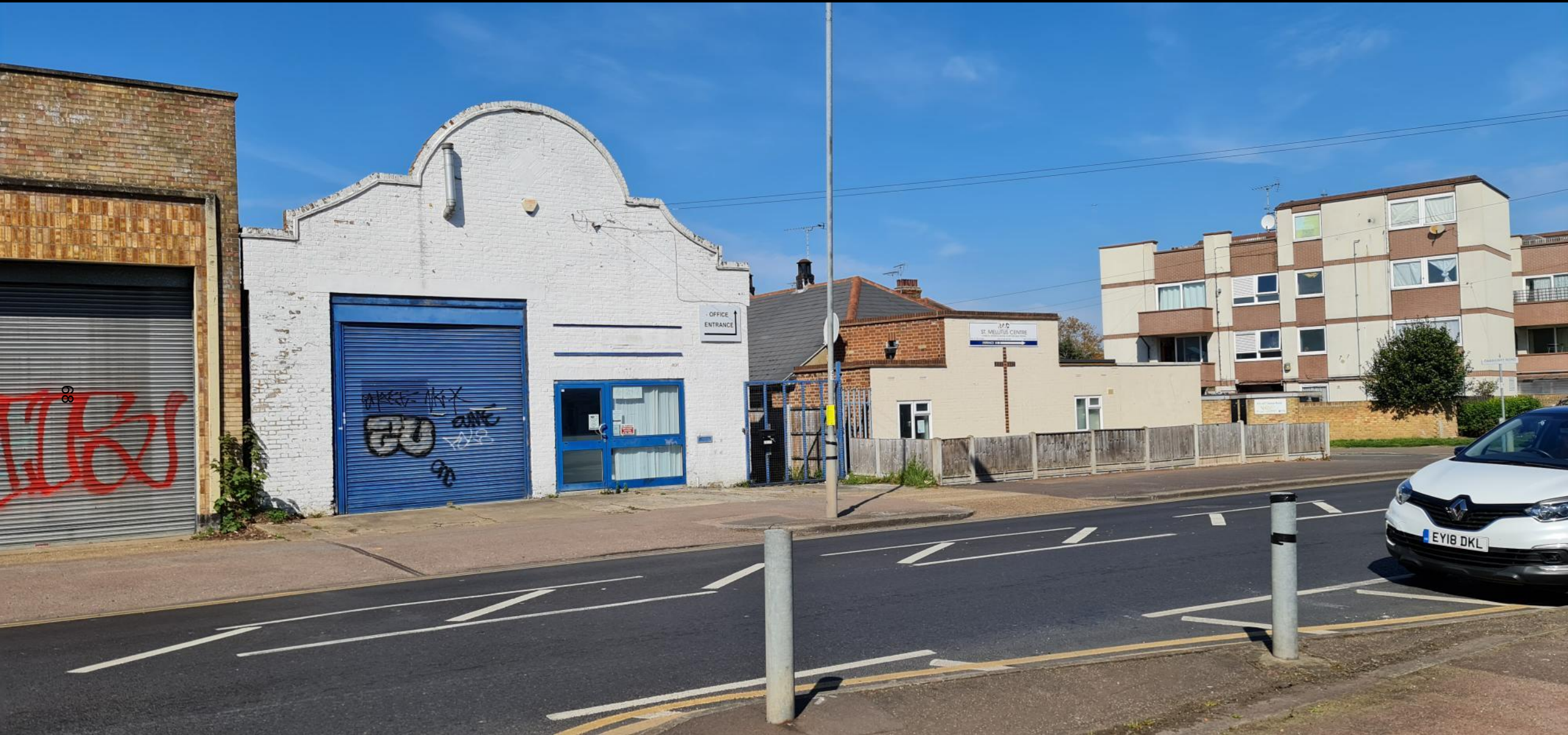
North end of site neighbouring St Mellitus Centre
