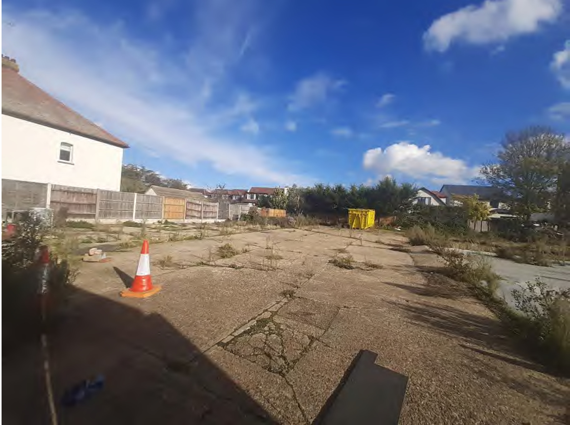
The application site
