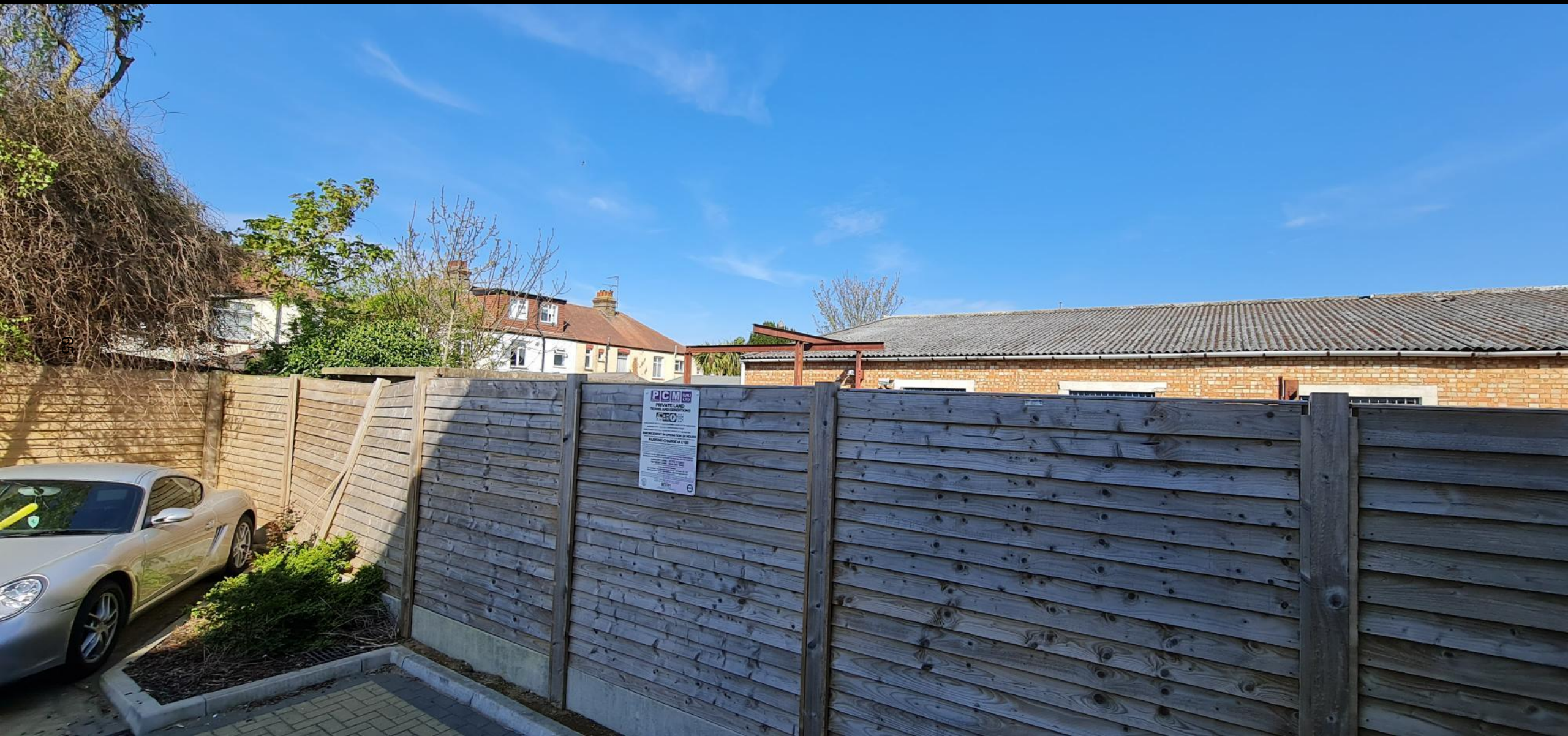
Site boundary with rear of Hammond Court; rear of neighbouring Glenhurst Road houses beyond
